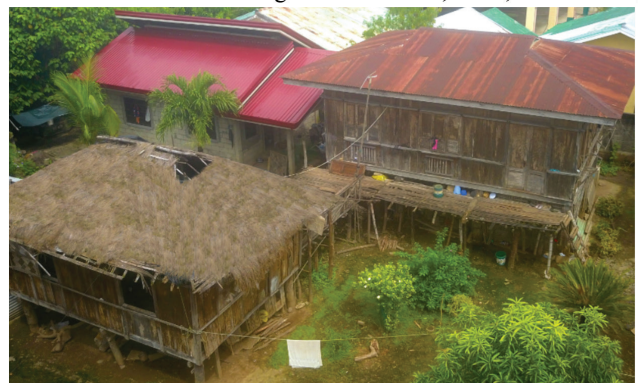
Figure 4: A modified version of the Itawes vernacular house but still maintaining the bridge or balag between the main house and the kitchen.
