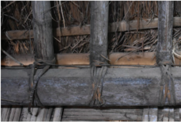
Figure 5: Rattan used as a knotting material.
