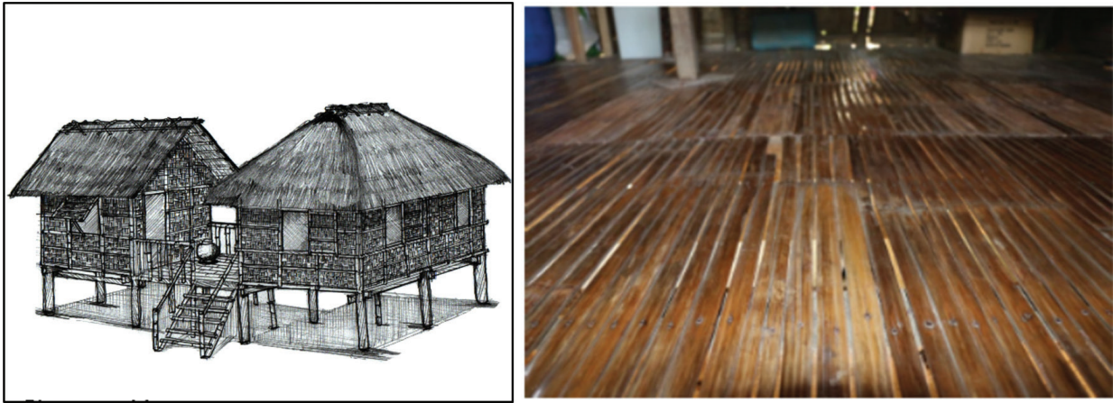
Figure 3: Researchers' impression of the Itawes House (left) and actual elevated flooring made of bamboo (right).
