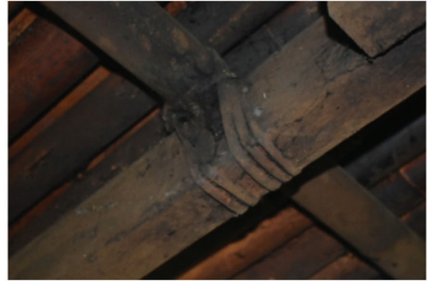
Figure 5: Rattan used as a knotting material.
