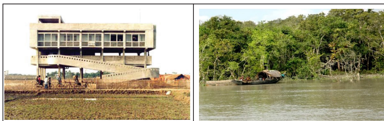
Figure 5. Disaster management via cyclone/flood shelter (left) and mangroves restoration (right). Mangroves can protect the coast against waves, currents and storms, and from coastal erosion. Mangroves can act as live sea walls and is more effective than concrete wall structures. Image source: https://www.google.com.au .
